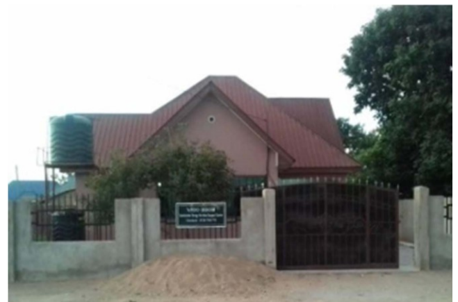
Figure 3: Sustainable Energy Service Support Centre (Dodoma)
