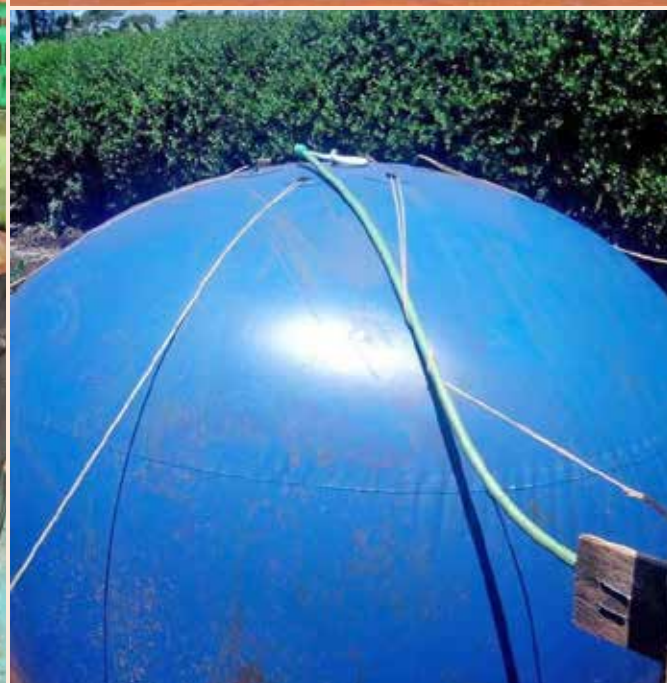
Photos: Takamoto biogas
