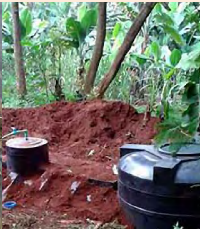
Photo: Blueflame Water and Energy Solutions
