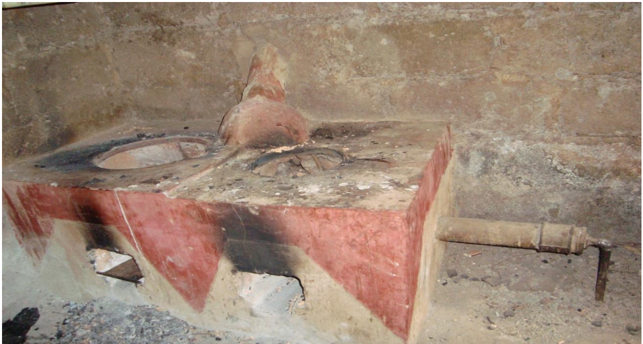
Figure f: Modified Okoa number 1 stove with metal pipe which direct hot/warm water to the bathroom (shower) or tap.
