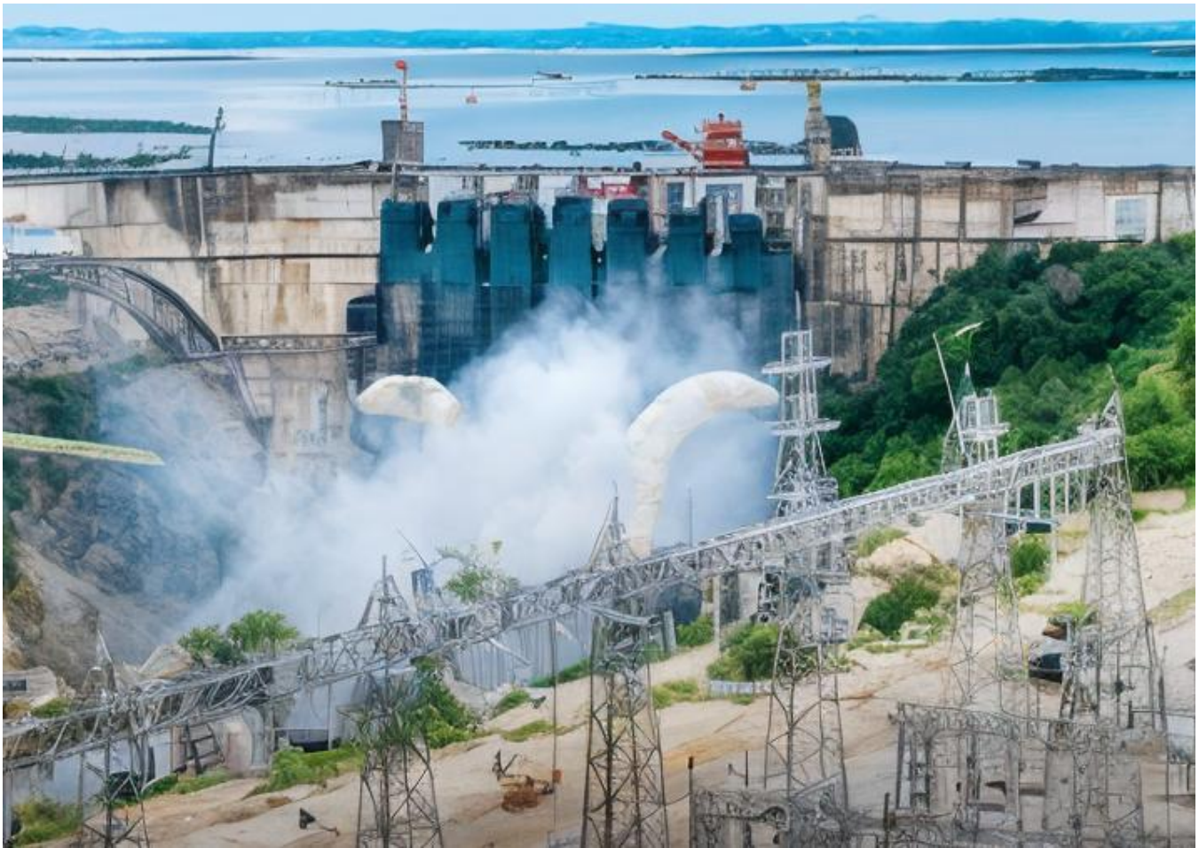
Mwalimu Nyerere Hydro Plant
